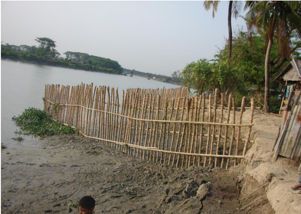
A view of bamboo bandalling for the protection of river bank
